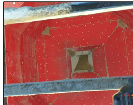
ABOVE K-Slide® UHMWPE Low Friction Liner installed in MS Bin.
