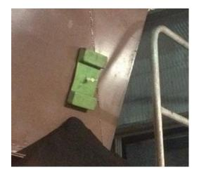
Our customer was able to resolve the leak immediately by applying the magnetic wear and repair K-Magnaplug®.
