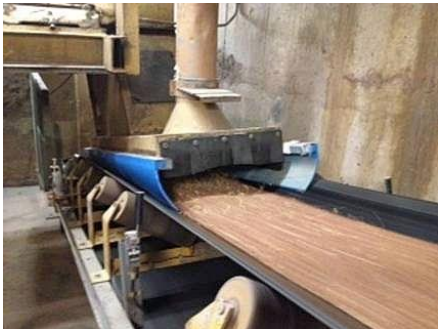
Photo of K-Snap-Loc® installed around the transfer point - the blue polyurethane indicates the Fire Resistant Anti Static FRAS properties.
