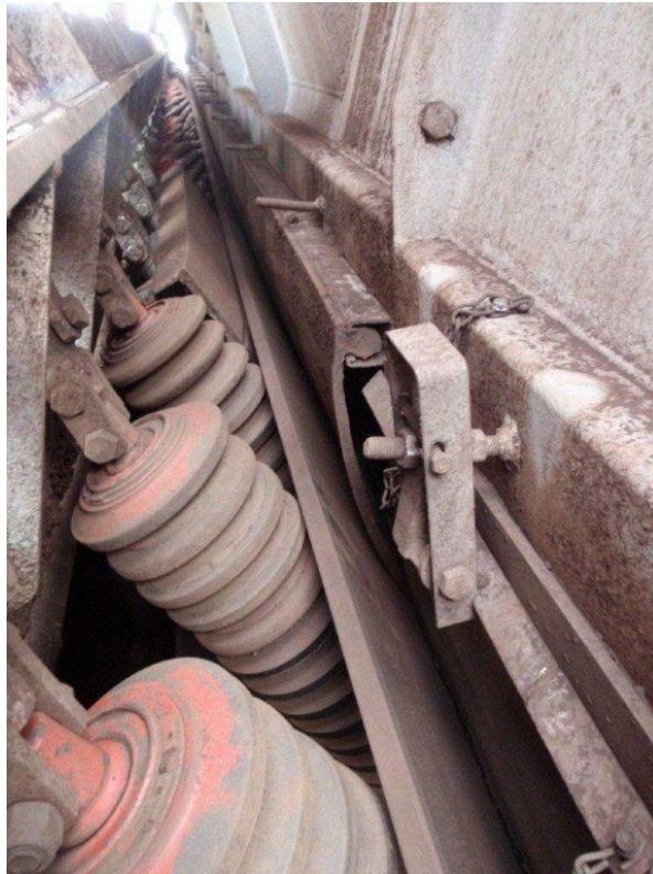
Photo taken February 2013 of K-Snap-Loc ® Dust Seal System in place on slider beds at Power Station, Traralgon, Victoria.
