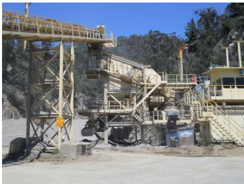
Above: photo of conveyor system showing chute and screen configuration.
